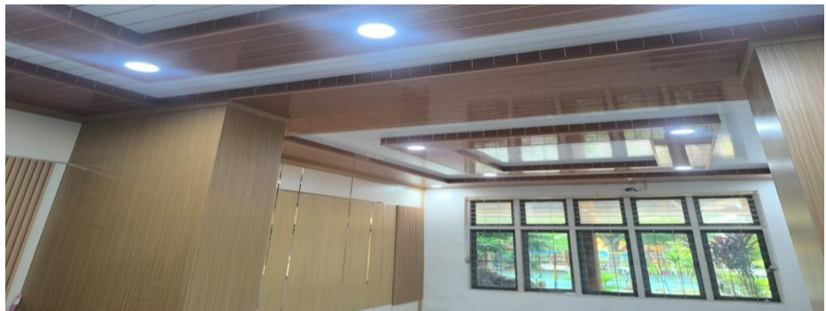
Gambar 3.5 Rehab Gedung SMA Lab School
